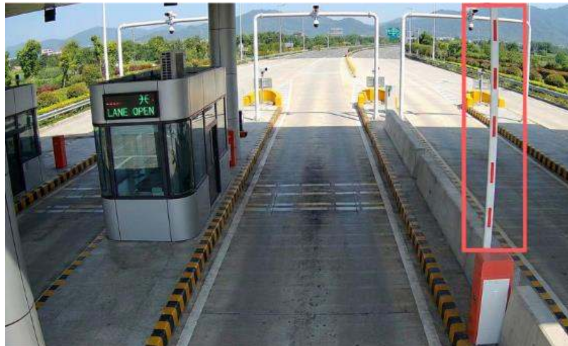
Barrier gate status monitoring
